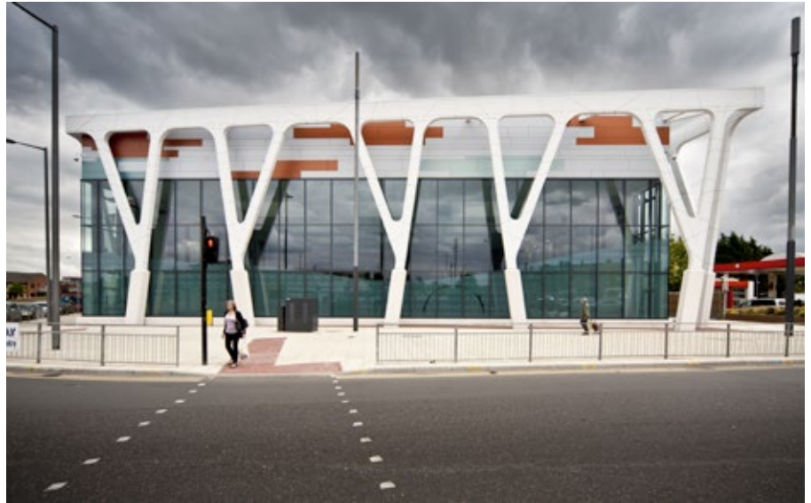
Becontree Heath Leisure Centre in Dagenham – the country's busiest pool
